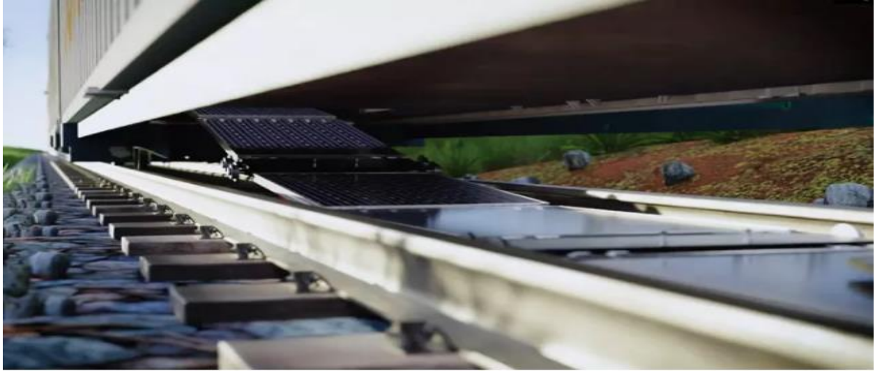
A specially designed train will unfurl the panels as it travels along the track. - Sun-Ways
